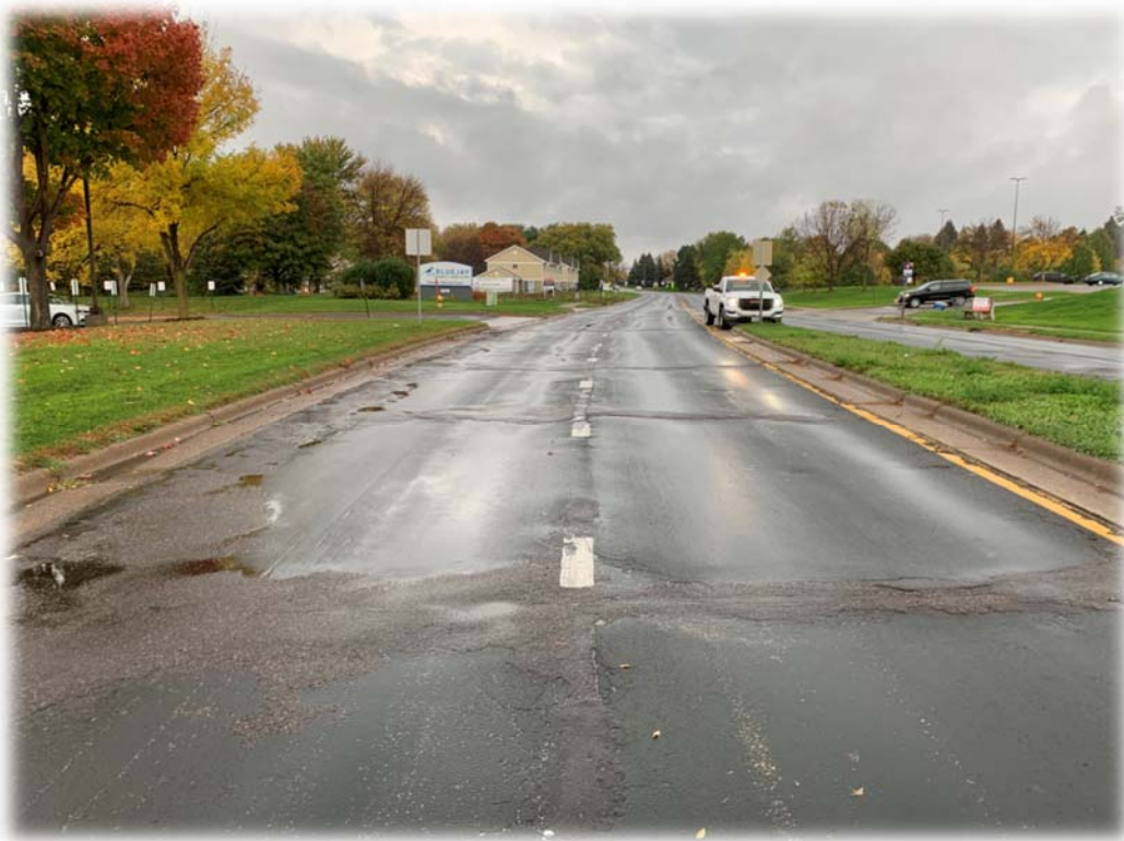
FIGURE 2: Photos of Pavement Deterioration in the Gervais Neighborhood
